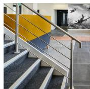
Using Gradus Grip adhesive for fixing down the Gradus GTX51 & GXT11 profiles at Humber Enterprise Project was more cost effective as it is quicker than mechanically fixing each nosing, it also shortened the installation time as the adhesive sets quicker so there is no need to shut the staircases off for long periods.
